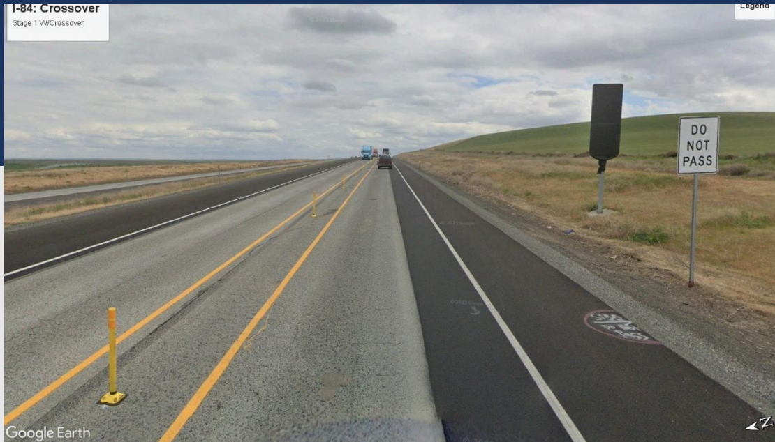
2-way, 2-lane traffic I-84 EB
