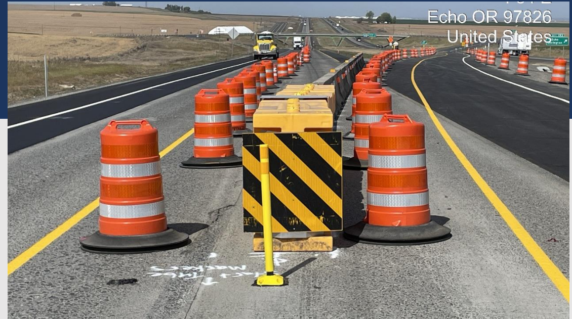
Traffic separated by barrier at crossover
