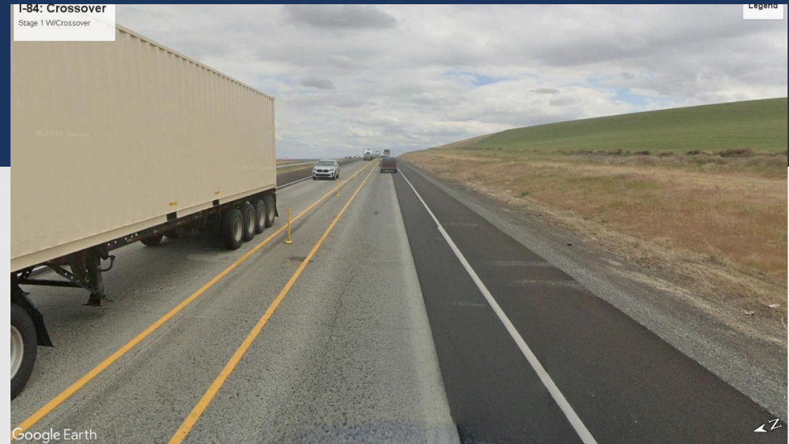
2-way, 2-lane traffic I-84 EB
