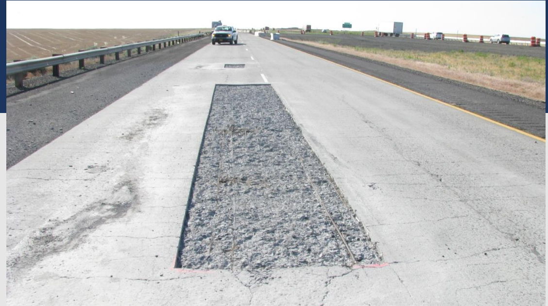
Spall repairs
