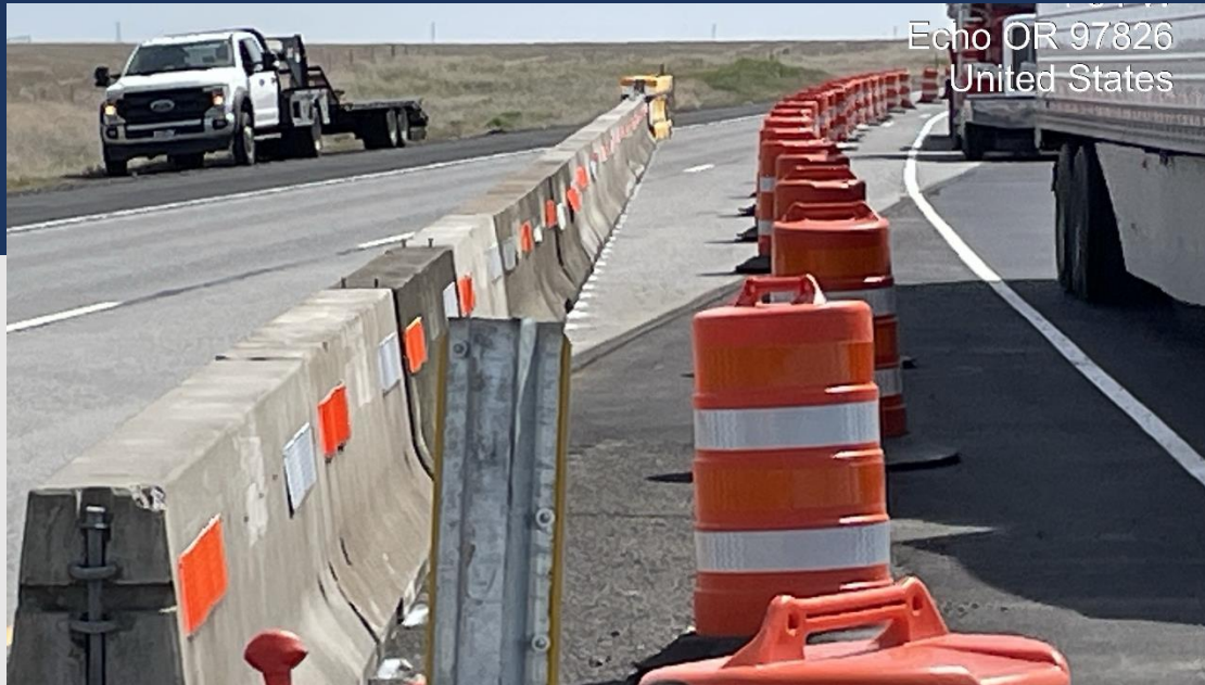
Work zone protected by barrier at traffic switch
