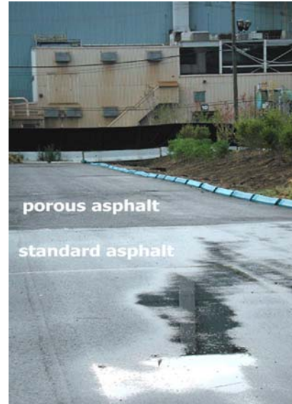
Figure 7.9 – Porous & Standard Lot Sections
