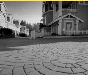
Colored and textured asphalt application using StreetPrint™
