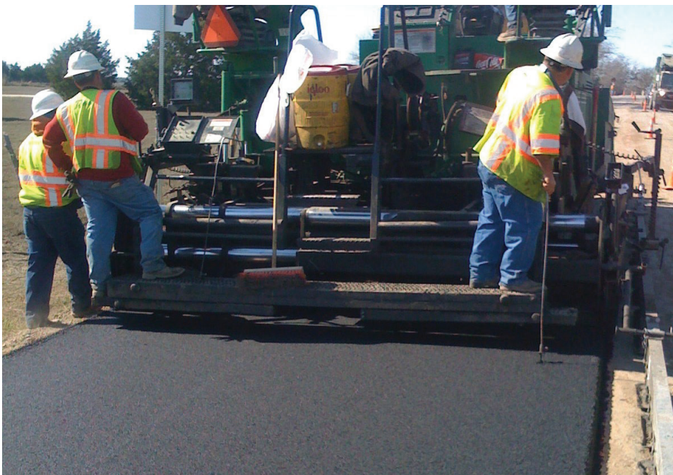
Figure 23. A Thinlay incorporating 40% RAP is used to restore ride quality to a rough PCC pavement.
