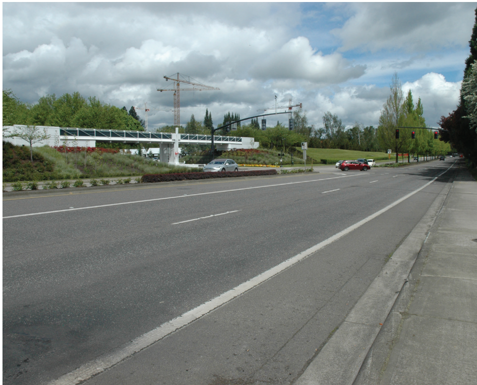
Figure 27. Thinlay placed in 2001; photo taken June 2017
