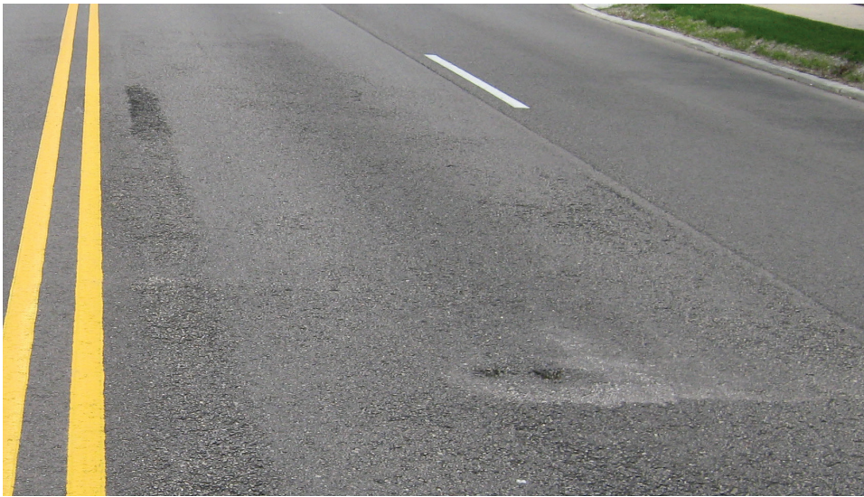
Figure 16. Slight raveling
