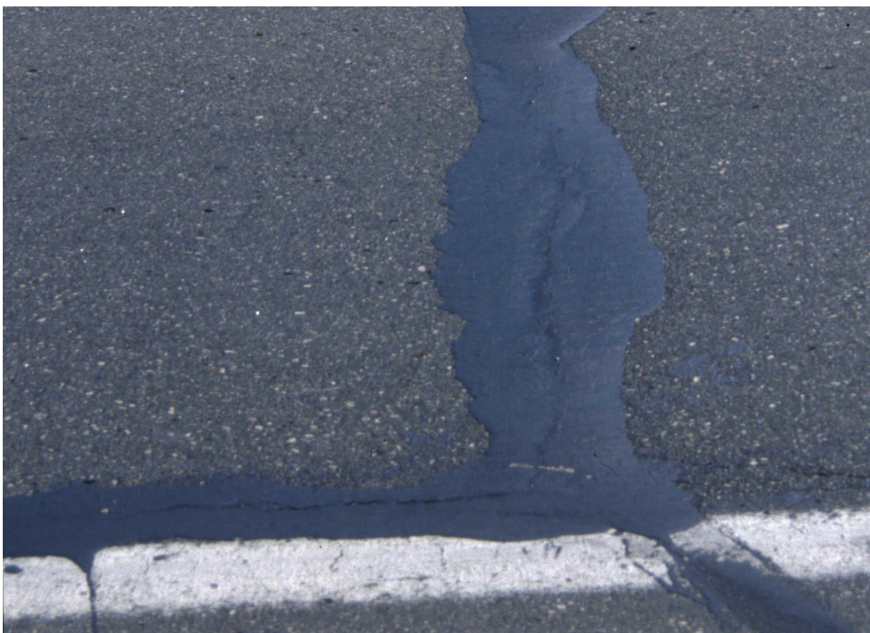
Figure 15. Overbanded crack sealing.
