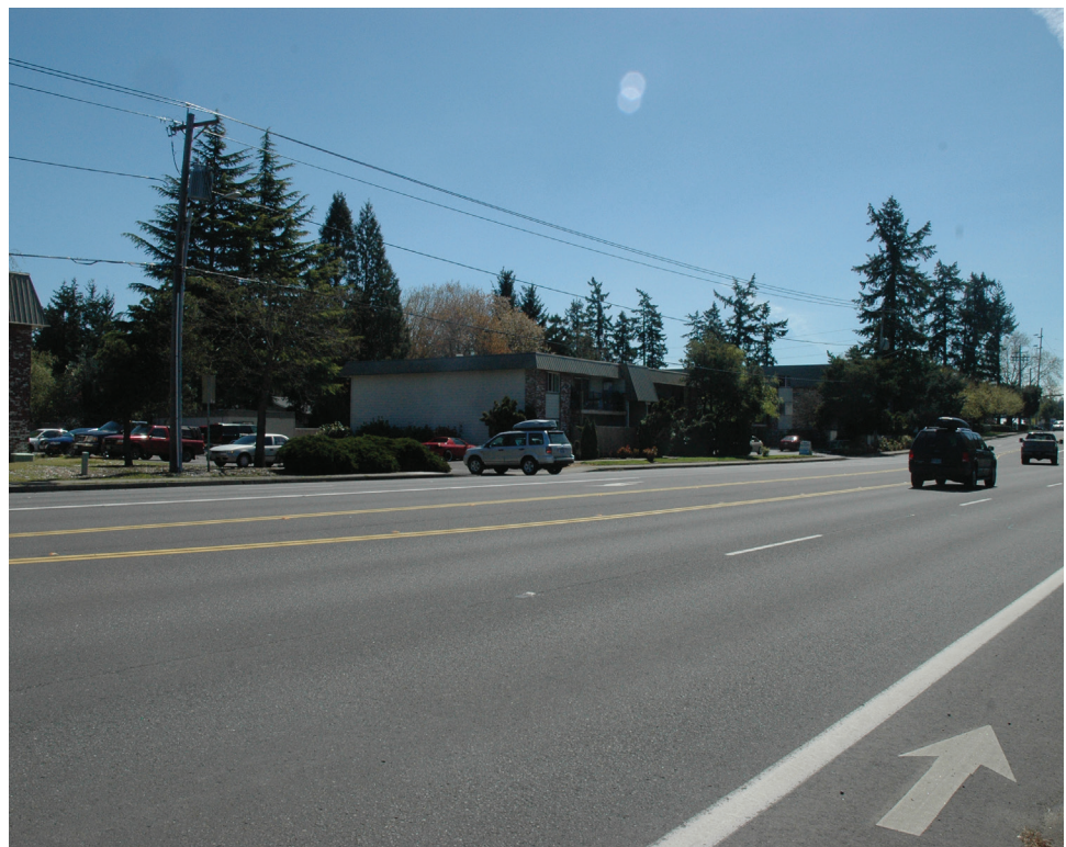
Figure 28. Thinlay placed in 2007; photo taken June 2017
