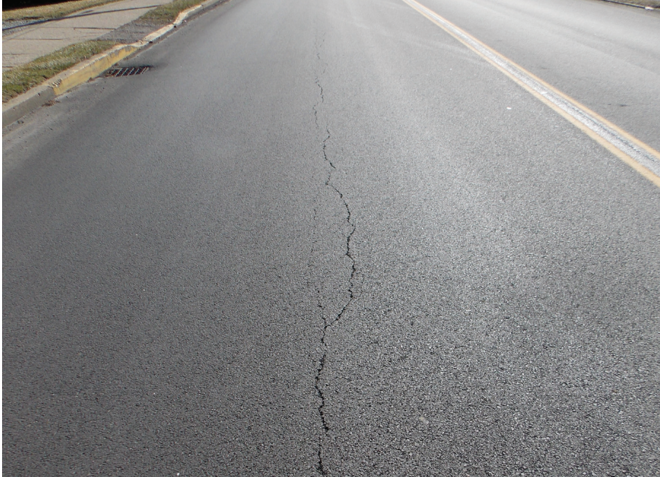
Figure 9. Longitudinal cracking
