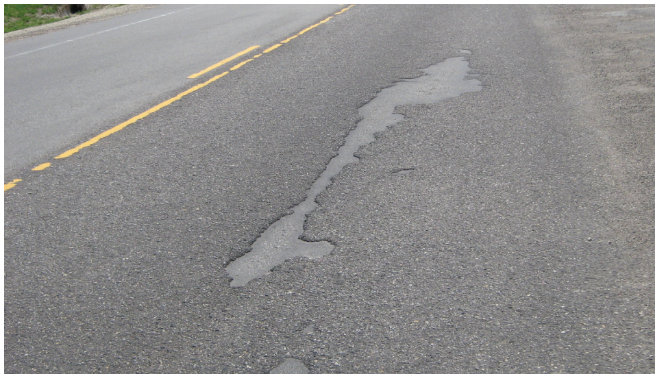
Figure 18. Severe raveling
