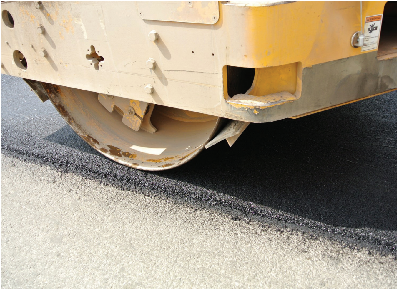
Compaction of a Thinlay mixture
