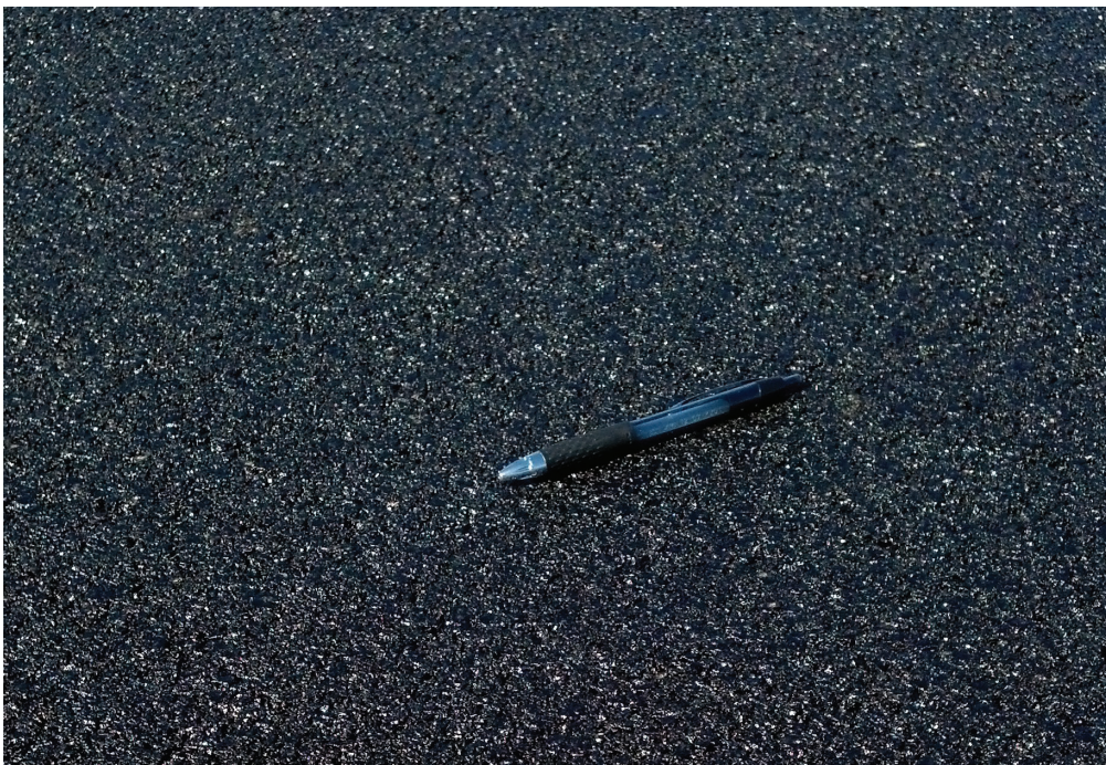
Figure 1. Dense Thinlay surface before compaction
