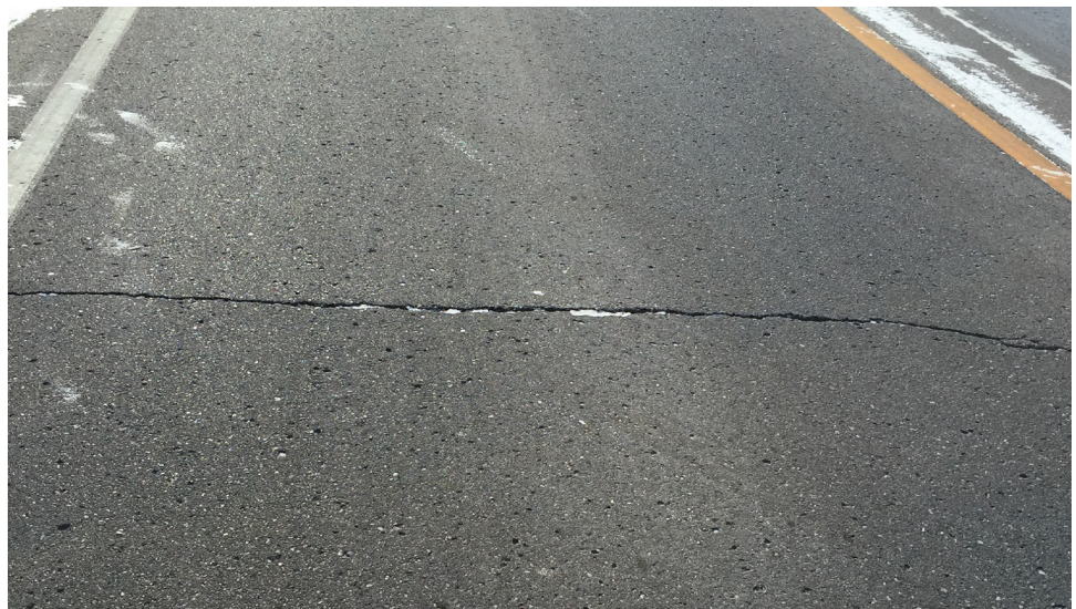
Figure 11. Thermal cracking
