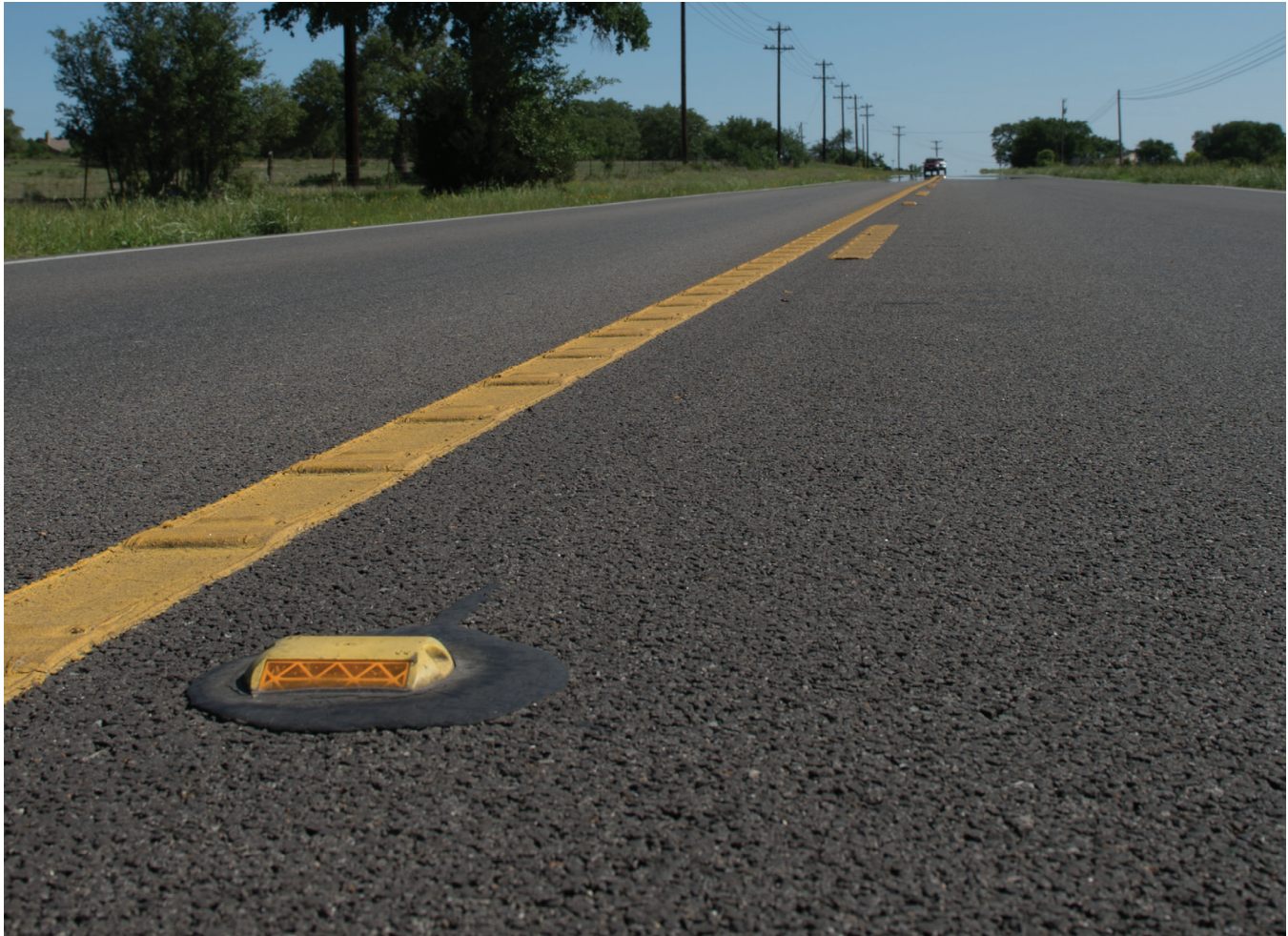
A Thinlay on RM 12 in Dripping Springs, Texas, helped significantly reduce road noise while also improving surface friction and thus safety.
