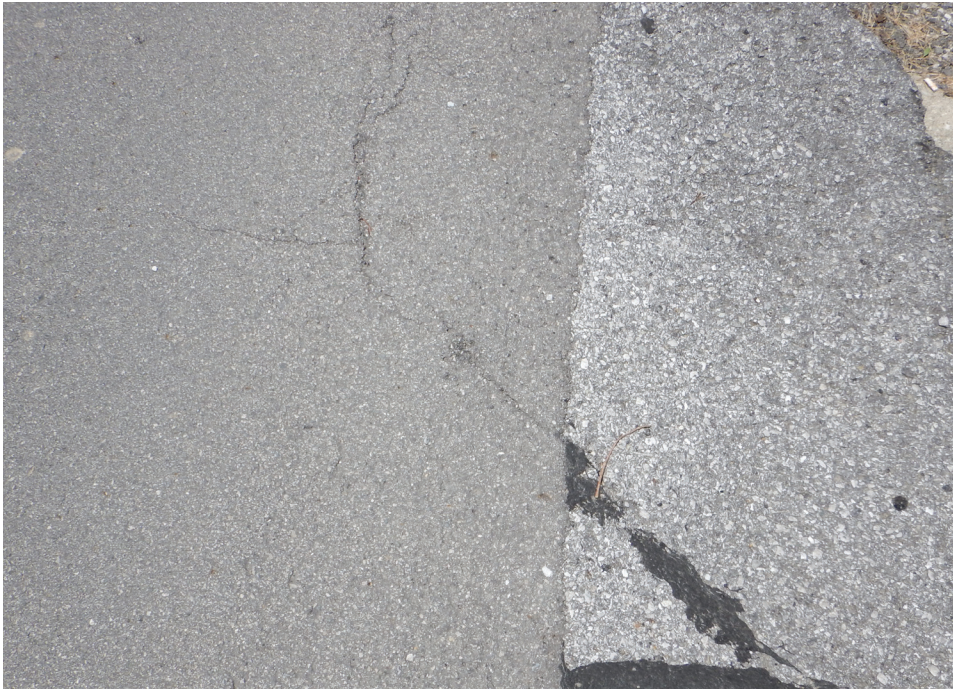
Figure 14. Reflective cracking
