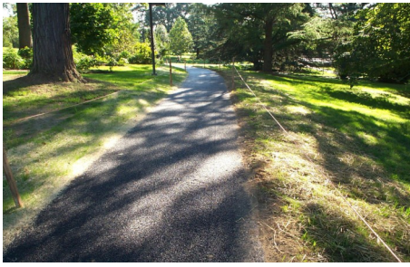
Figure 7.10 – Porous Asphalt Walking Paths
