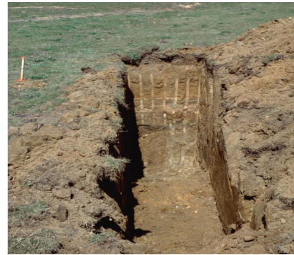
Figure 7.7 – Deep Hole Excavation
