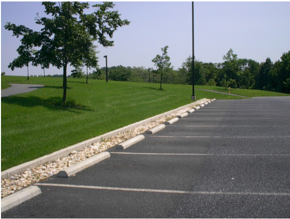
Figure 7.6 – Repaved, Unpaved Stone Edge
