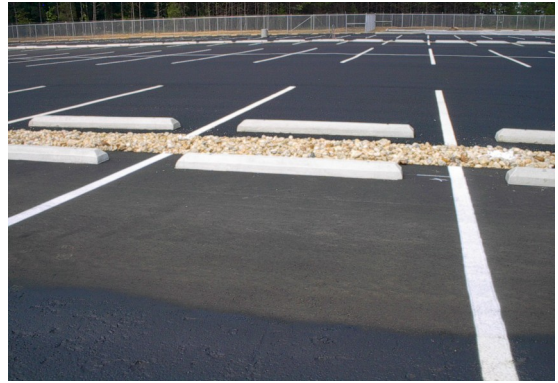
Figure 7.12 – Large Commuter Parking Lot
